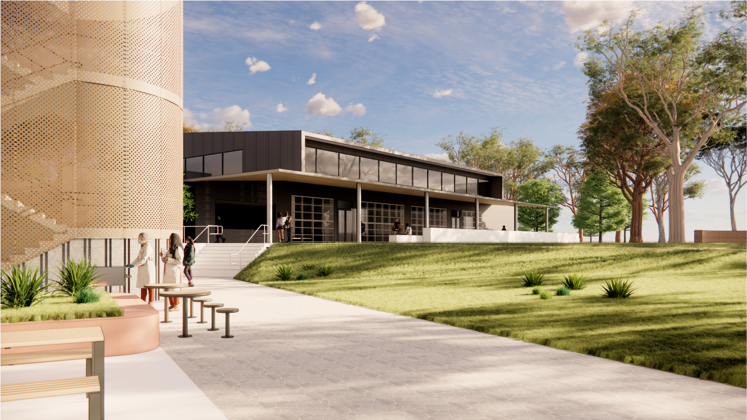
View from Block C looking at Gymnasium
